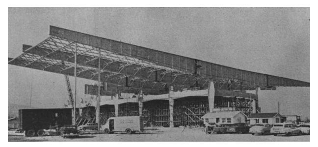
Plate 45. Skidmore, Owings & Merrill. Cantilever construction for United Airlines hangar, San Francisco International Airport. *Engineering News-Record*. 30 January 1958.
