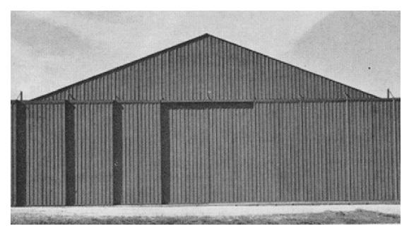
Plate 54. Butler Manufacturing. Prefabricated hangar for the Army Air Forces, with steel doors and roof. 1945. *The Military Engineer*. May 1945.
