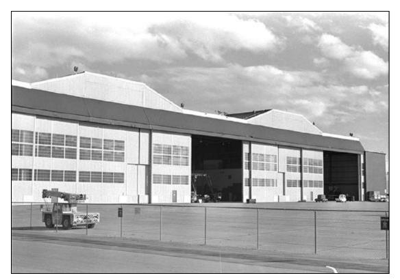
Plate 24. Mills & Petticord. Double-cantilever hangar at Kirtland Air Force Base. View of 1998. Photograph, K.J. Weitze.
