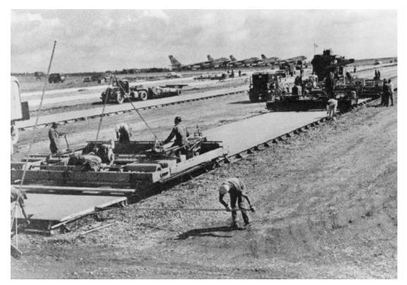
Plate 85. Original aphaltic concrete paving at Loring Air Force Base. 1948. Reproduced from Army Engineers in New England (1978).
