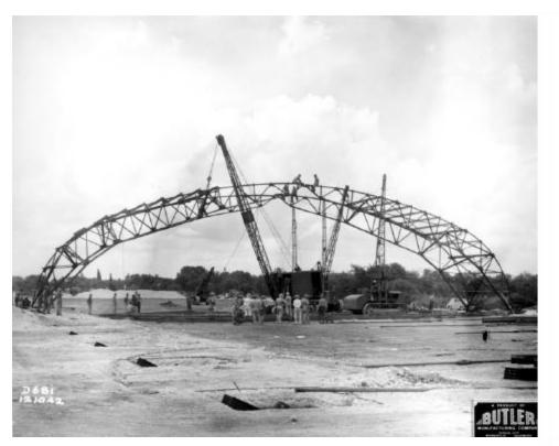
Plate 50. Butler Manufacturing. Erection of the superstructure for the canvascovered hangar, Army Air Forces. 1942. Courtesy of the Butler Manufacturing Company.
