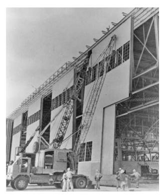
Plate 40. Construction for recessing doors. Doublecantilever hangar program. Courtesy of Kuljian Corporation.
