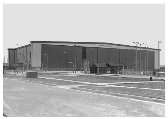
Plate 129. Renovated double-cantilever hangar. Whiteman Air Force Base. (Identical changes at McConnell and Shaw Air Force Bases.) July 1999. Photograph, K.J. Weitze.
