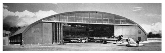
Plate 5. Dyckerhoff & Widmann. Thin-shell concrete hangar completed outside the U.S. Reproduced from *The Military Engineer*, January-February 1940.
