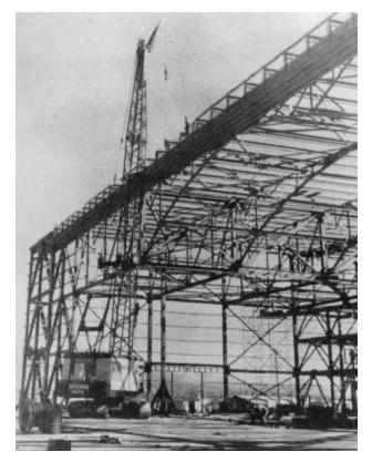
Plate 39. Double-cantilever hangar under construction at March Air Force Base. *Engineering News-Record*. 12 May 1955.
